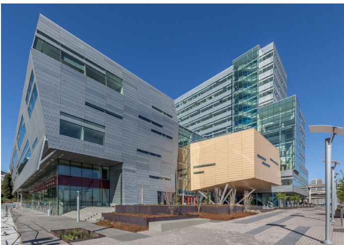
The Collaborative Life Sciences Building houses health and science programs for OHSU, PSU and OSU.
